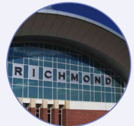
Richmond International Airport recently underwent a complete renovation and expansion.
